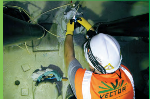
Post-Tech® PTI Impregnation System used to mitigate corrosion in post-tensioned bridge
