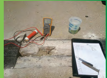
Corrosion potential testing
