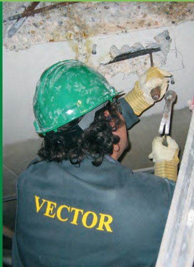
Inspection of test excavation and screwdriver penetration test
