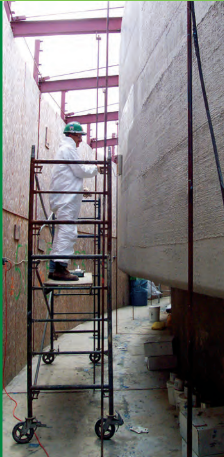
Coating installation over FRP strengthening system on a post-tensioned structure
