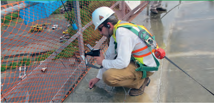
Borescope inspection on post-tensioned tank tendons
