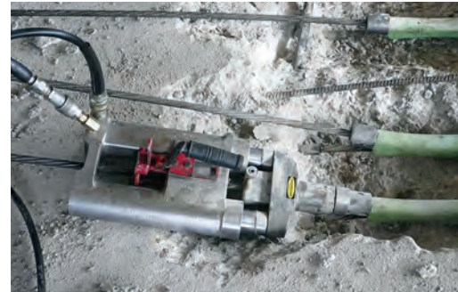
Post-tensioning repair using center stressing chuck
