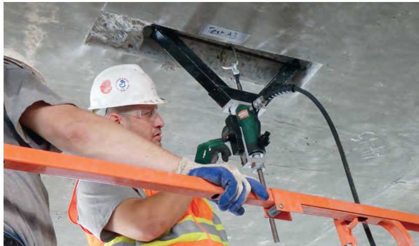
In-situ tension testing
