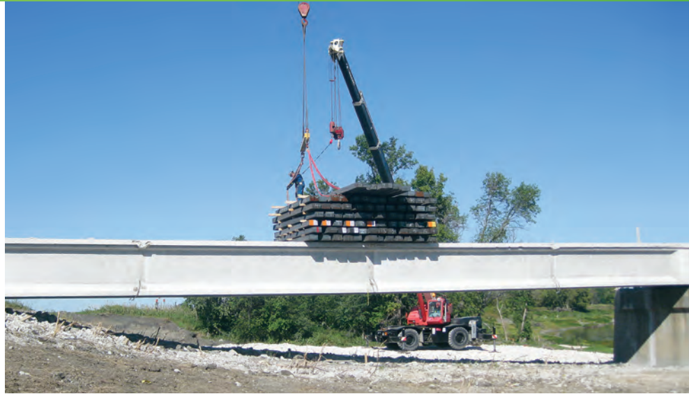
Instrumented load testing of post-tensioned bridge girder
