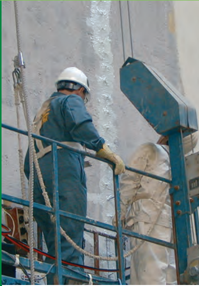
Epoxy injection of cracks in post-tensioned containment structure
