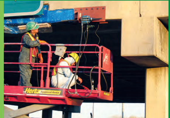
Installation of external post-tensioning system to strengthen damaged bridge girder
