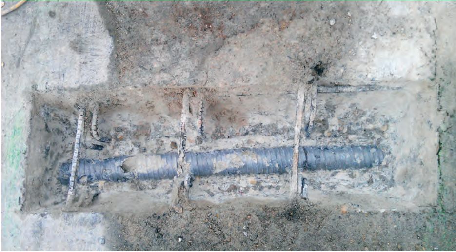
Inspection of grouted (bonded) post-tensioned tendon
